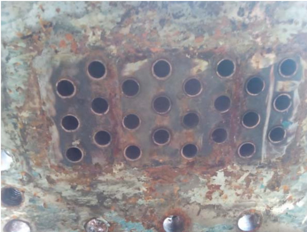
AFTERCOOLER BEFORE CLEANING
